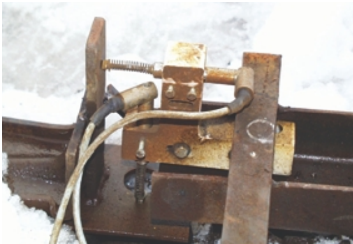
Displacement transducers for measuring horizontal and vertical components in track displacement on a curve
