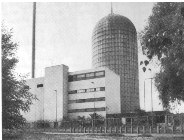
Fig. 1: The HDR Test Facility in Karlstein am Main
