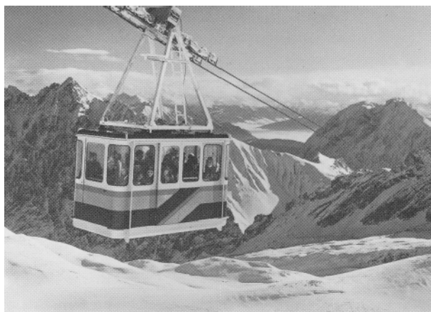
Fig. 1: The cablecar system, with two track cables and one hauling cable is ideal for short, steep grades such as this one with maximum track grade of about 30 deg
