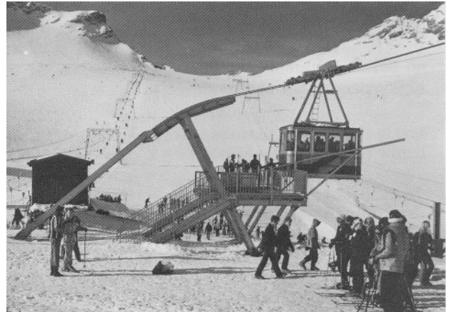
Fig. 2: View of bottom station with platform for boarding cablecar reveals its simple and relatively inexpensive design
