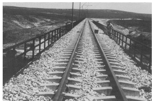
Fig. 7: View of the rails and concrete sleepers imbedded in crushed stone ballast
