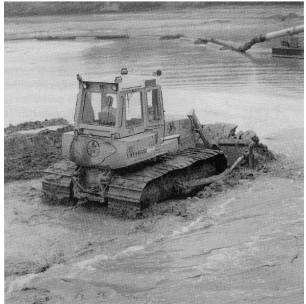
Fig. 1: Bulldozer in operation on ground covered by water.
