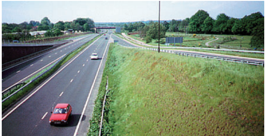
Fig. 1: The green "outer skin" of a synthetics-reinforced support structure on a motorway in England
