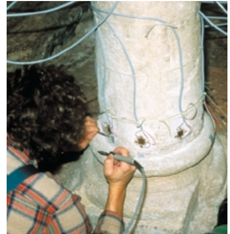
7c: Installation work at the foot of the column
