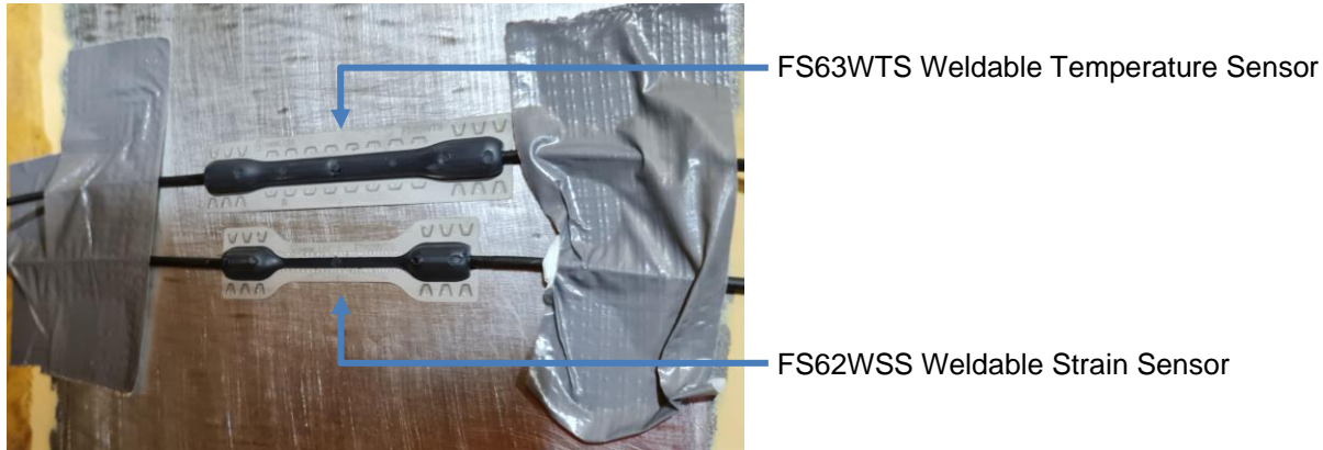
Figure 3 Installed weldable strain and temperature sensors
