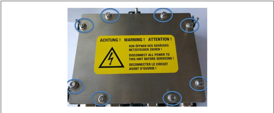
Fig. 21.2 Unscrew the nuts at the marked points.
