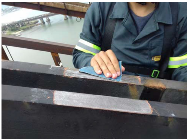
図2.3 溶接面の研磨
