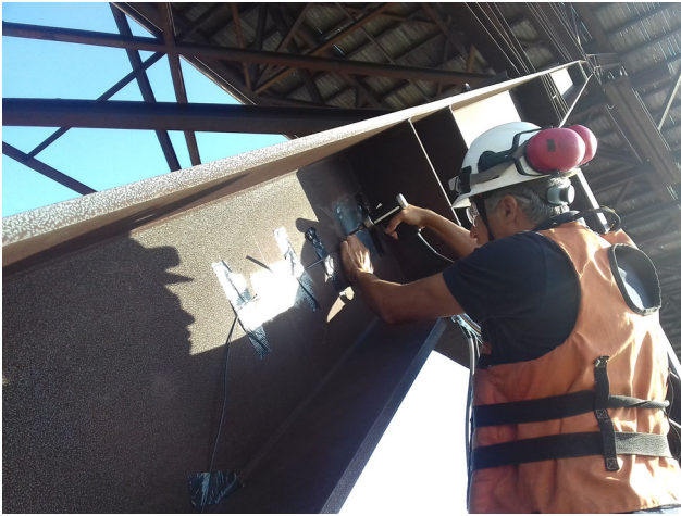
Fig. 2.17 Welding the sensor
