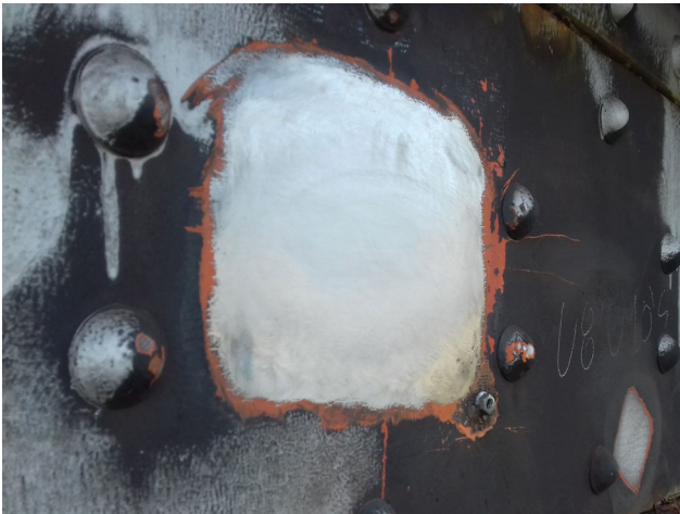
Fig. 2.4 Ready to weld surface
