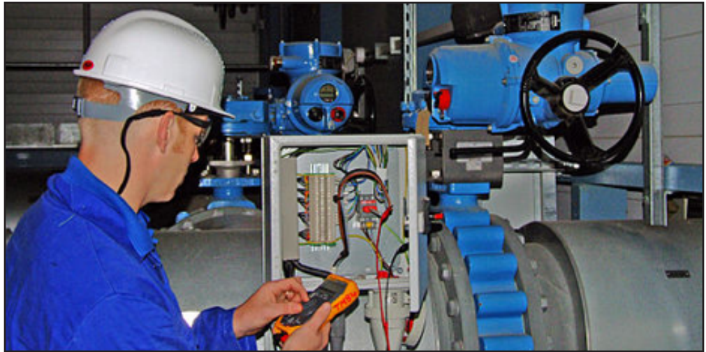
Figure 1. Three-phase drives, like the one shown here, are taking the place of mechanical actuators in many industrial applications.
