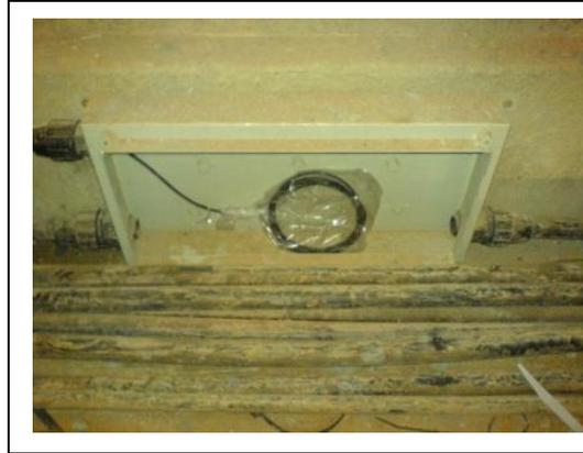
Fig. 37: Optical cable connection box
