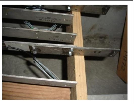
Fig. 28: Mechanical connection between bars
