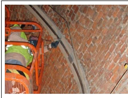
Fig. 35: Tightening of the pre-supports
