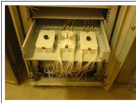
Fig. 39: Optical cable connection to the rack
