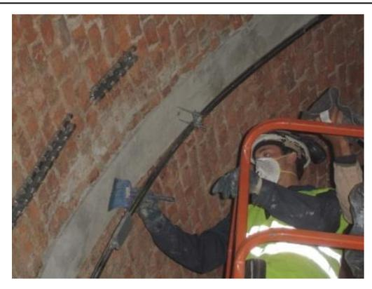
Fig. 32: Cleaning of the surface
