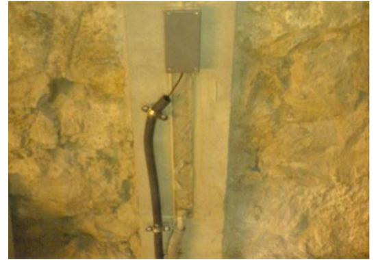
Fig. 38: Jumper protection
