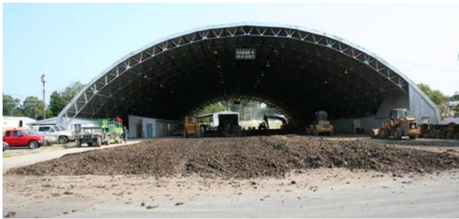
Fig. 2. At 375 feet long and 145 feet wide, the ERDC Pavement Testing Facility is big enough to allow construction, traffic testing, and analysis of several test sections at once. It also includes offices for Carr and Brogdon, as well as storage space for construction materials, tools, equipment, and data acquisition instrumentation.
