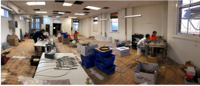
Figure 7. System assembly works.
