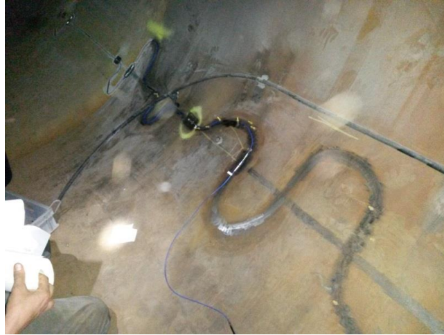
Fig. 9: Installation of sensors in section-type B
