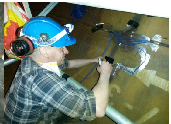
Fig. 18: Cleaning the surface with alcohol
