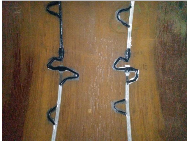
Fig. 7: Installation of sensors in section-type A
