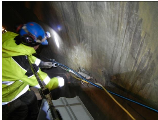
Fig. 23: Fixing the flexible tube to the stainless steel support cable
