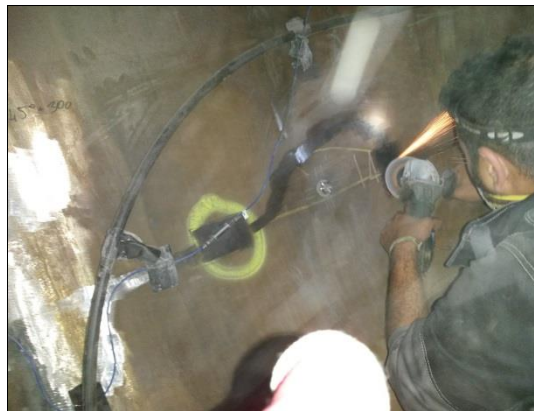
Fig. 17: Deburring the surface
