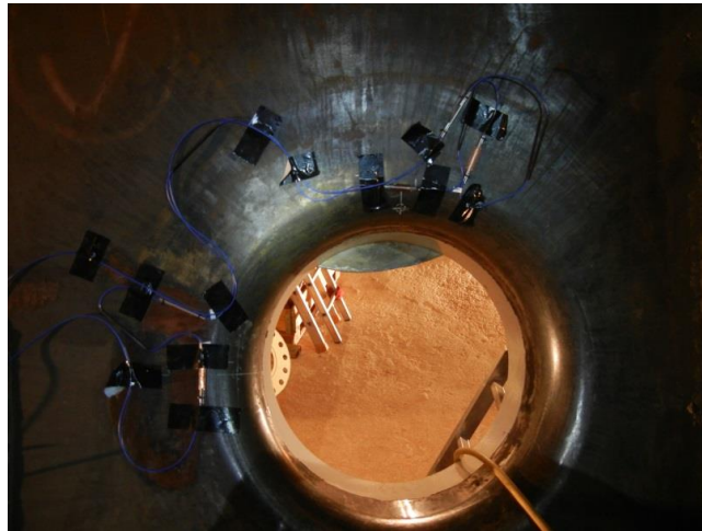
Fig. 11: Installation of sensors in section-type S
