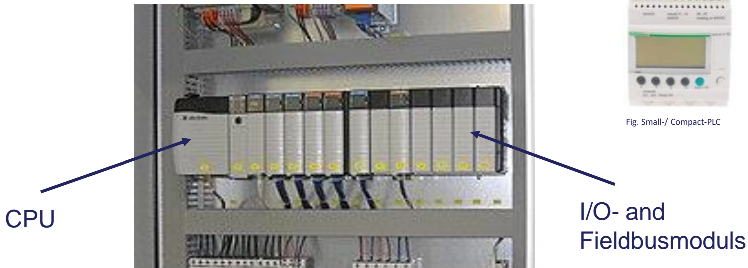
Fig. Control cabinet with PLC consisting of CPU (head station) and peripheral I / O modules
