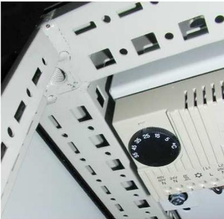
Fig. 2.8 Temperature controller.
