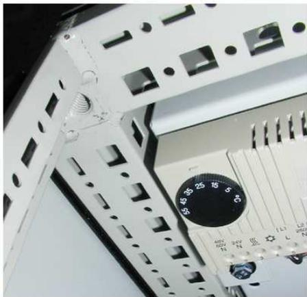
Fig. 2.6 Temperature controller.
