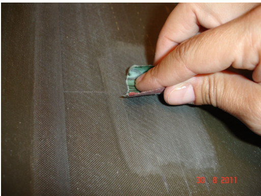
Fig. 2.2 Sanding the surface to remove remaining paint or rust
