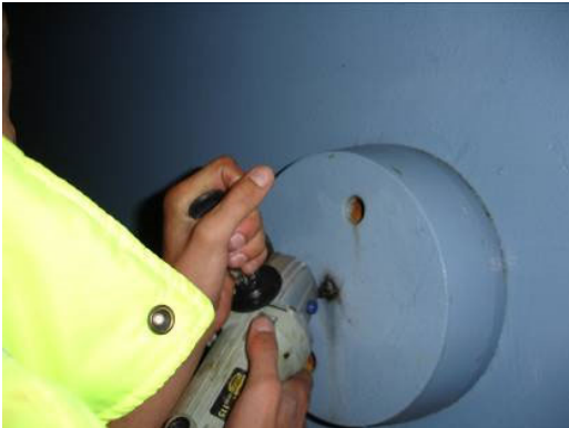
Fig. 2.1 Deburring the surface to remove paint or rust
