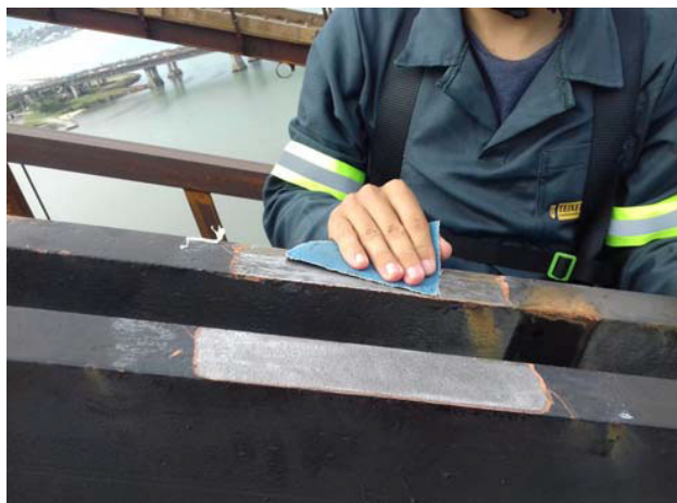
図2.4 溶接面の研磨
