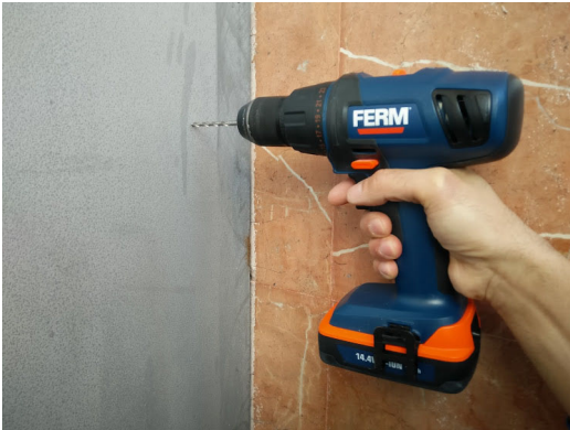
Fig. 2.4 Drilling the fixation holes
