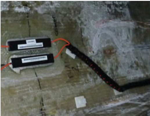
Fig. 2.8 Cable protected with corrugated tubes
