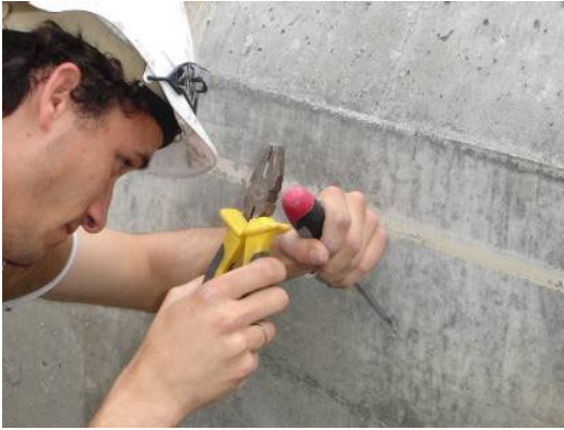
Fig. 2.1 Removing irregularities from the surface
