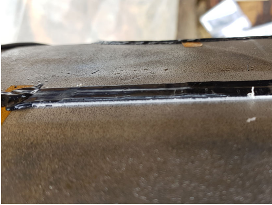
Fig. 2.15 Gluing area after removing the tape.
