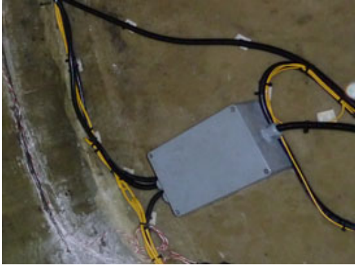
Fig. 2.8 Protection boxes for extra cable and connections
