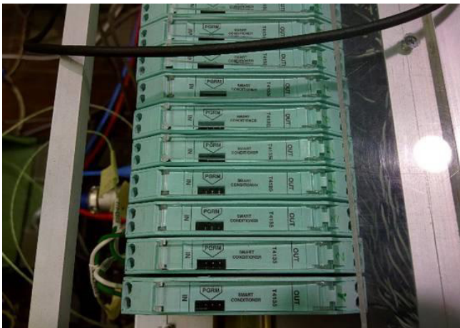
Fig. 4.a: Programmable isolation amplifiers for temperature measurement
