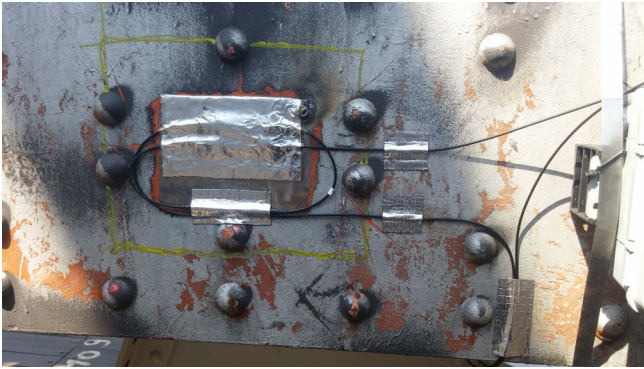
Fig. 2.33 Sensor protected with ABM75
