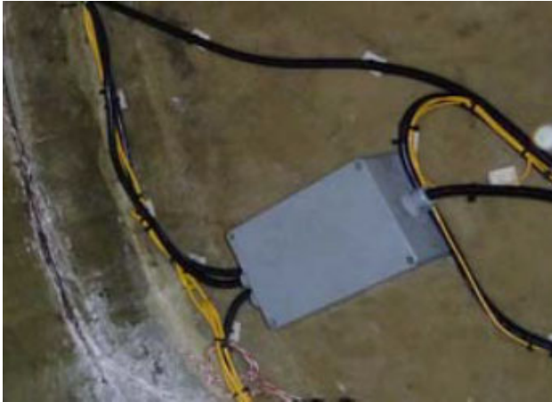
Fig. 2.31 Protection boxes for extra cable and connections
