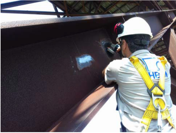
Fig. 2.1 Surface deburring
