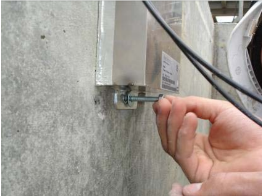
Fig. 2.5 Applying the washers and hexagon nuts
