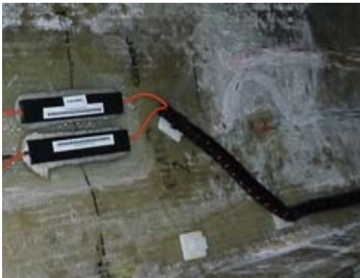
Fig. 2.14 Cable protected with corrugated tubes
