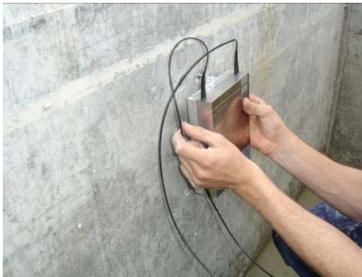
Fig. 2.4 Placing the sensor on the supports
