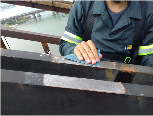
図2.3 溶接面の研磨
