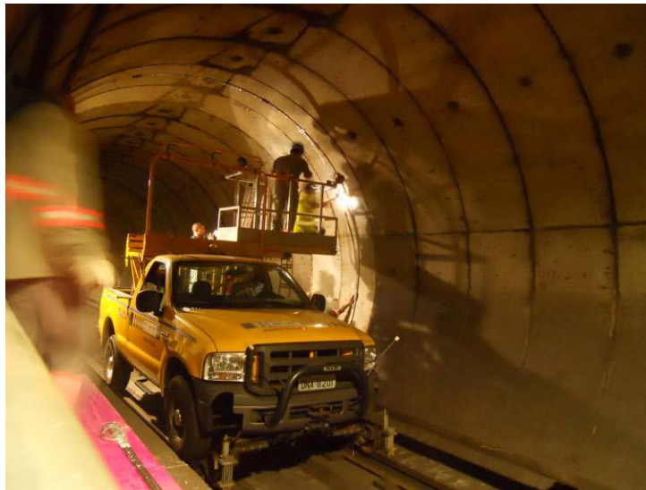
Figure 3. Installation of a measuring section for tunnel monitoring.
